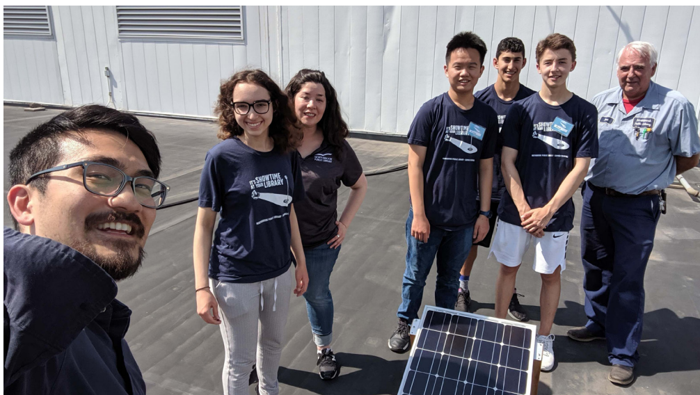
Teen volunteers help install a solar panel on the library's roof.
