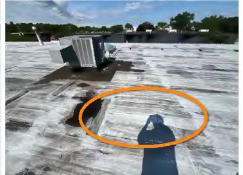
Center Of Watehouse Roof- Repair
