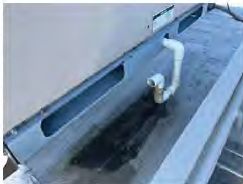
Upper Roof- Repair
