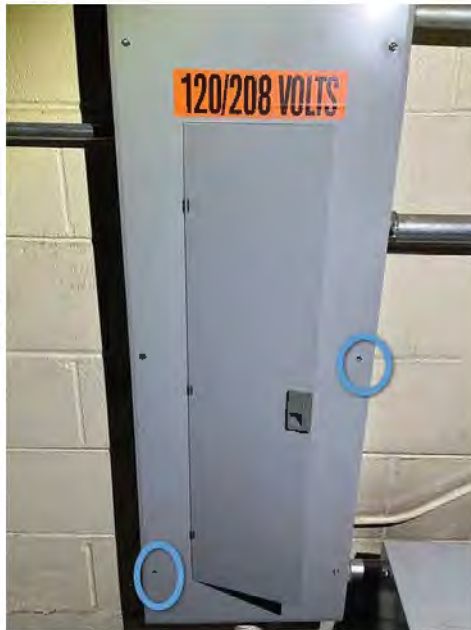
West Warehouse- Replace
