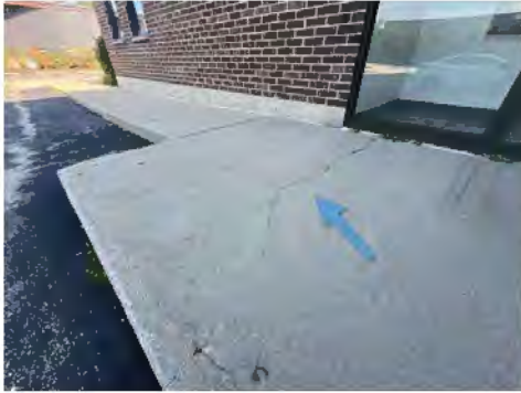
South Entrance- Repair
