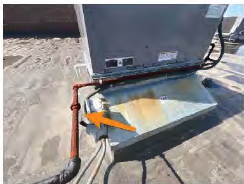
Lower Roof HVAC Unit 1- Replace
