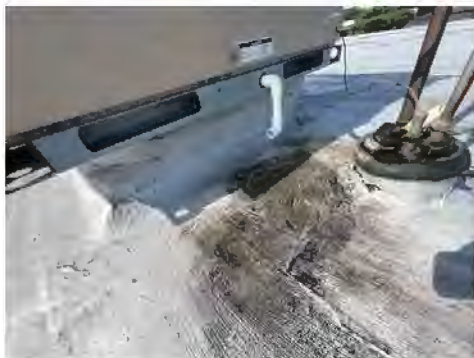
Upper Roof- Repair
