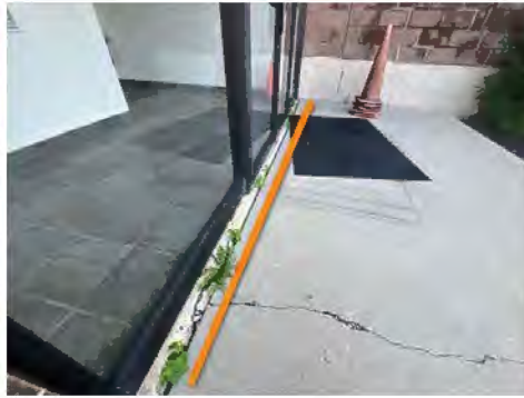
Southwest Entrance- Repair
