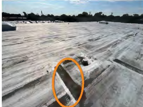
Center Of Watehouse Roof- Repair
