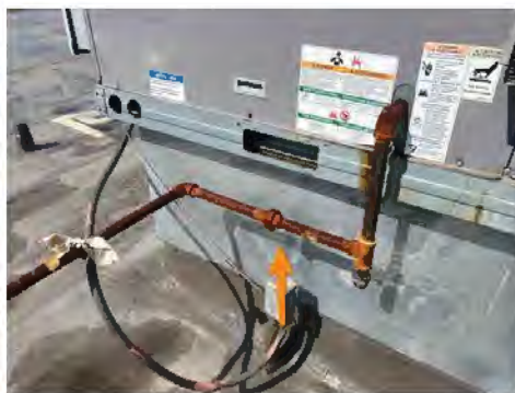
Lower Roof HVAC Unit 3- Replace
