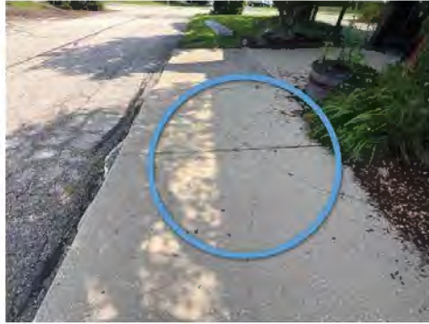
Main Entrance- Repair
